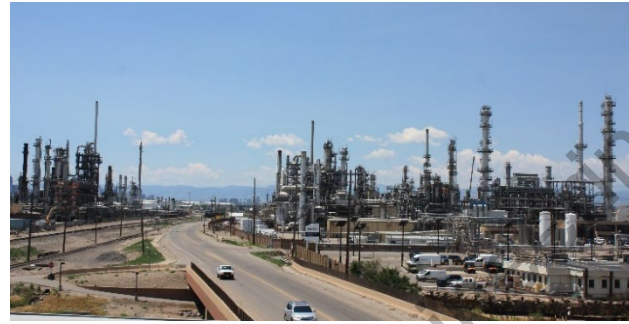
I-270 southbound looking southwest (passenger view) toward Brighton Blvd from Brighton Blvd overpass; Suncor refinery, Sand Creek, and Brighton Boulevard.
