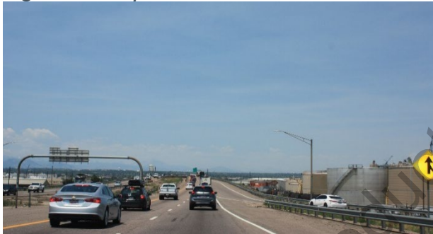
I-270 northbound looking northwest toward Vasquez Boulevard on-ramp. Industrial storage tanks at right, Suncor refinery to the left out of the frame.
