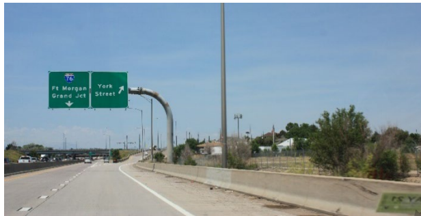
Northbound York Street off-ramp looking northwest. Welby Reservoir to right, residential area on slight hill below signs.
