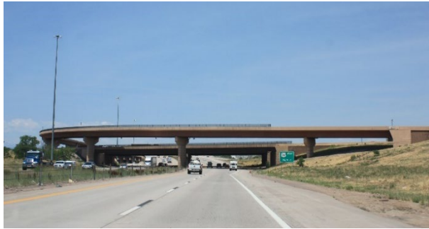
Northbound I-270 south of I-76 overpass looking northwest.
